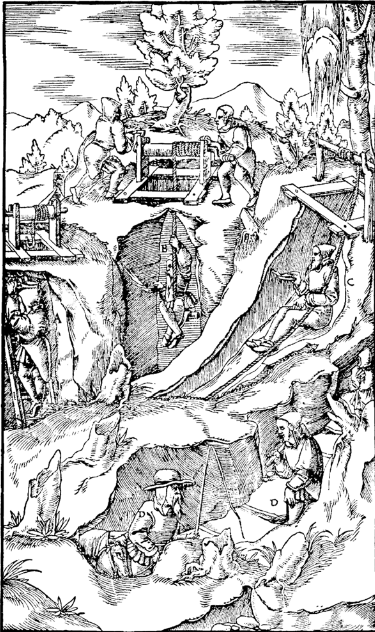
A—DESCENDING INTO THE SHAFT BY LADDERS. B—BY SITTING ON A STICK. C—BY SITTING ON THE DIRT. D—DESCENDING BY STEPS CUT IN THE ROCK.
