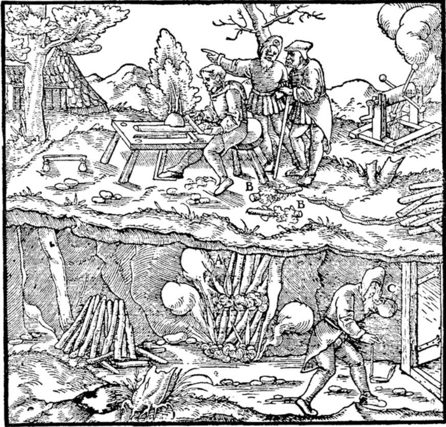
A—KINDLED LOGS. B—STICKS SHAVED DOWN FAN-SHAPED. C—TUNNEL.
