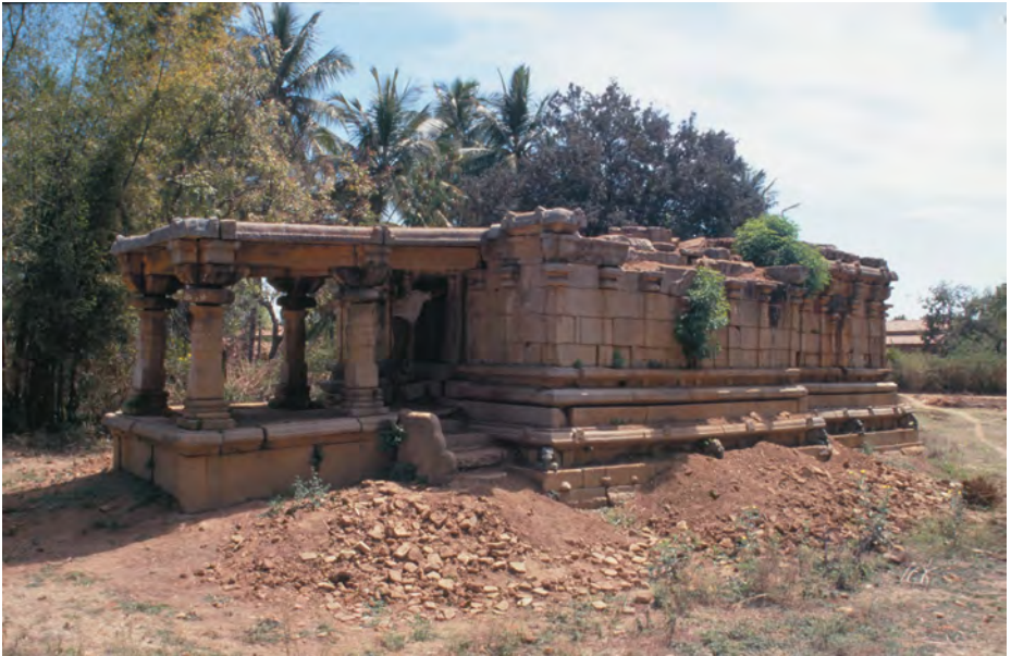
Fig. 6: External view onto the severely damaged former Pārśvanātha Jaina Temple at Hale Belgola, which has not been reconsecrated.
