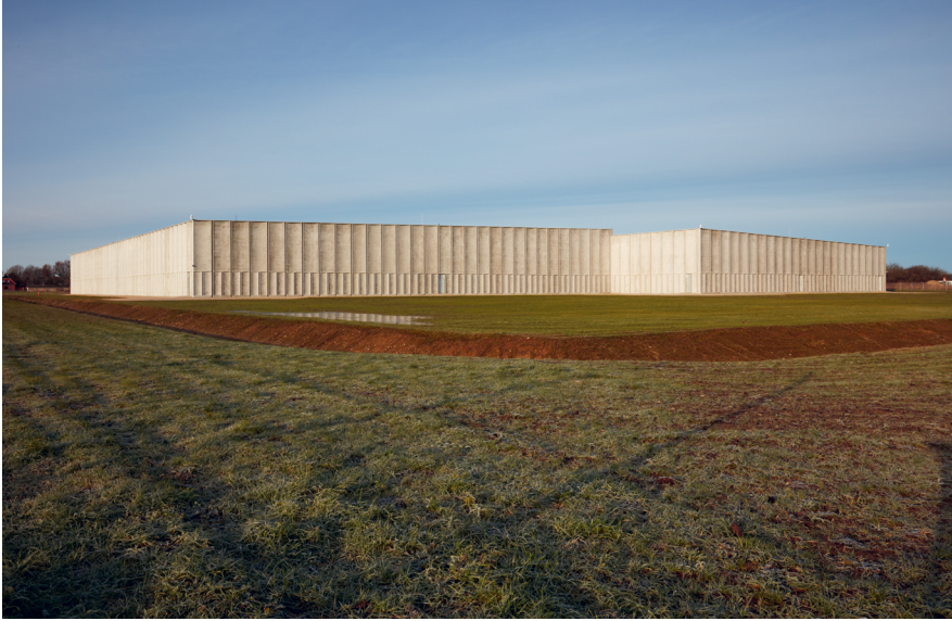
Fig. 4: The new storage was ready for moving in collections in 2022. Photo: Atle Clausen
