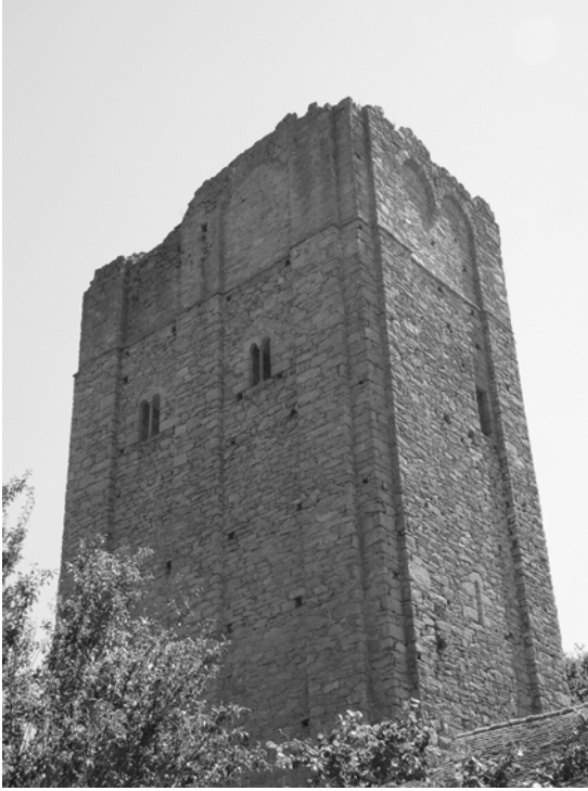
Figure 6: A Limousin tower that survives in original form and nearly full height: Chateau Chervic (French “Château-Chervix”, department of Haute-Vienne), built for the viscounts of Limoges in the later twelfth or early thirteenth century. Exterior 12.9 x 9 m, height nearly 30 m. Photo: Jadith Iacelle, 2022, for Wikimedia Commons.
