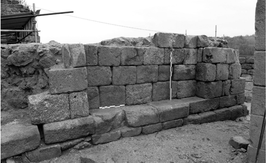
Figure 5: Ashlar of the square tower at Ventadorn (c. 1050–1150). Exterior of the northwest wall viewed from the courtyard. On the left is a central buttress, on the right, the buttress encasing a corner. Photo: L. D’Agostino during the archaeological campaign of 2005–2006.
