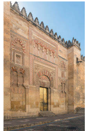
Fig. 4.10: Córdoba, Mezquita, Portal on the east facade restored by Ricardo Velázquez Bosco and the sculptor Mateo Inurria after 1908. Photo: Cornelia Steffens, 2015.
