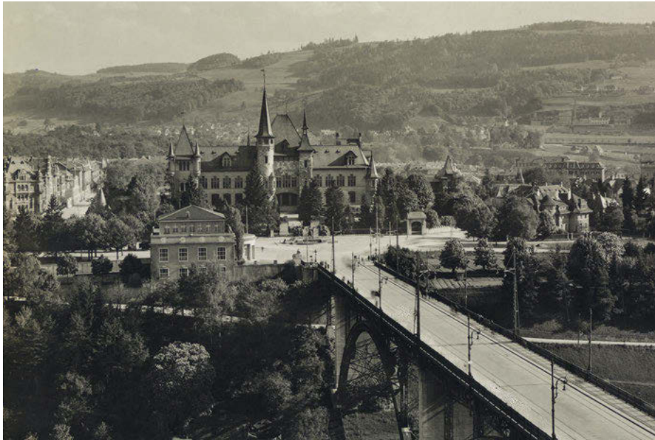
Fig. 11.1: View of the BHM from the Kirchenfeld Bridge, ca. 1927. Photo: ETH-Bibliothek Zürich, Bildarchiv, PK_005791 (public domain).
