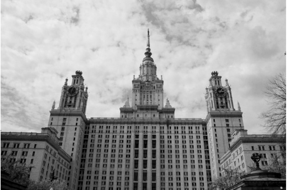
Fig. 2.9: M.V. Lomonosov, Moscow State University, 1949–53, one of the “Seven Sisters” buildings. Photo: Lynn Greyling (CCO public domain).
