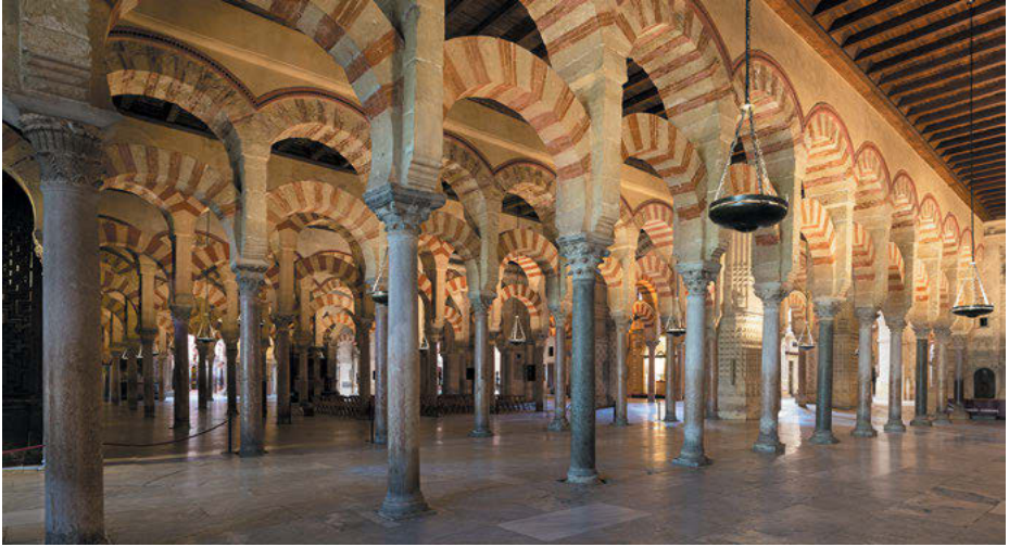
Fig. 4.2: Córdoba, Mezquita, Interior view toward the piers of the crucero from the northwest. Photo: Cornelia Steffens, 2015.
