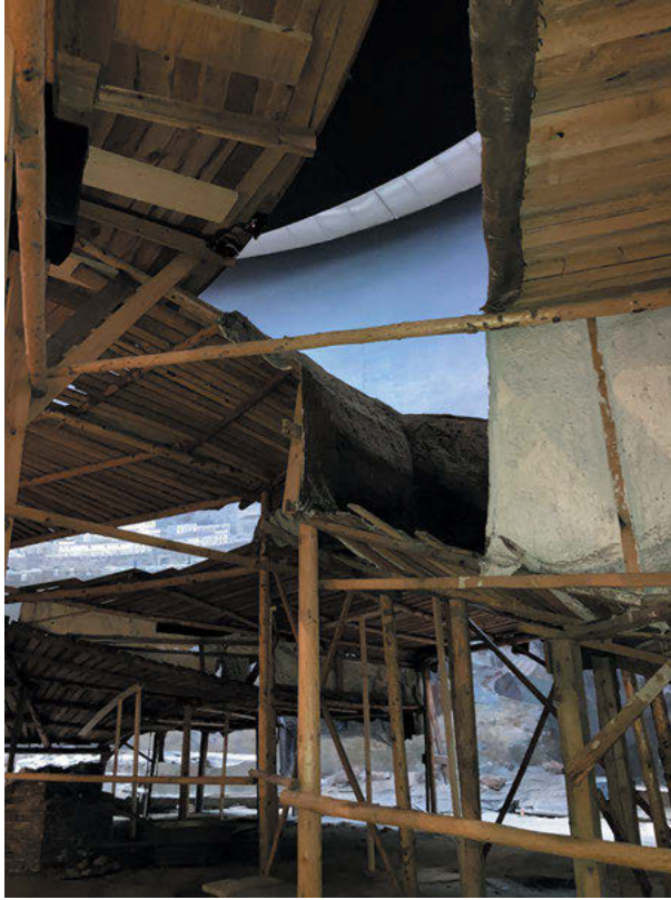
Fig. 3: Substructure of the faux terrain built with simple wooden slats, canvas and plaster. Image, the author.
