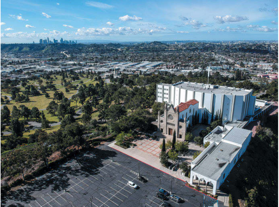
Fig. 4: Gothic-style entrance hall to Hall of Crucifixion-Resurrection, center right. The white cross, lit at night, can be seen widely from areas north of downtown Los Angeles. Image, James Fishburne, CC-BY-SA-4.0.
