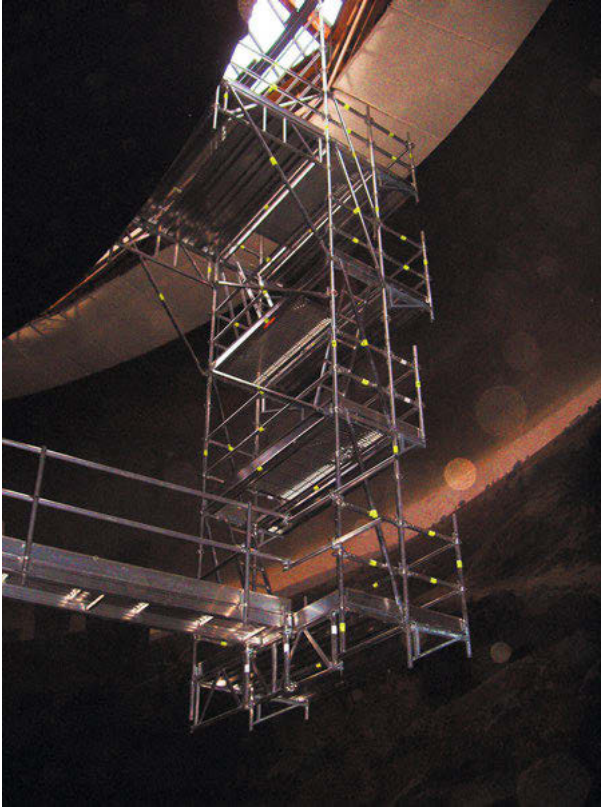
Fig. 4: Suspending light-weight scaffolding. Image, the author.
