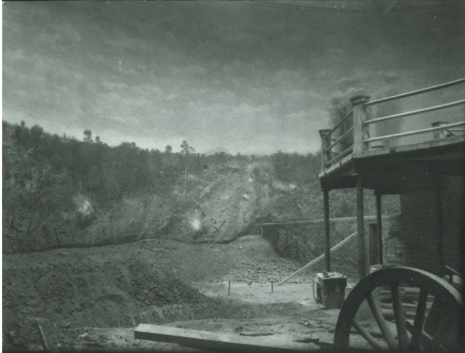
Fig. 3: The Battle of Atlanta's seventh faux terrain under construction in its “permanent” steel and brick building in Grant Park, 1935. Image, Atlanta History Center.
