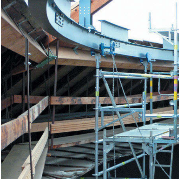
Fig. 5: Suspending light-weight scaffolding; mounting ring at the top. Image, the author.
