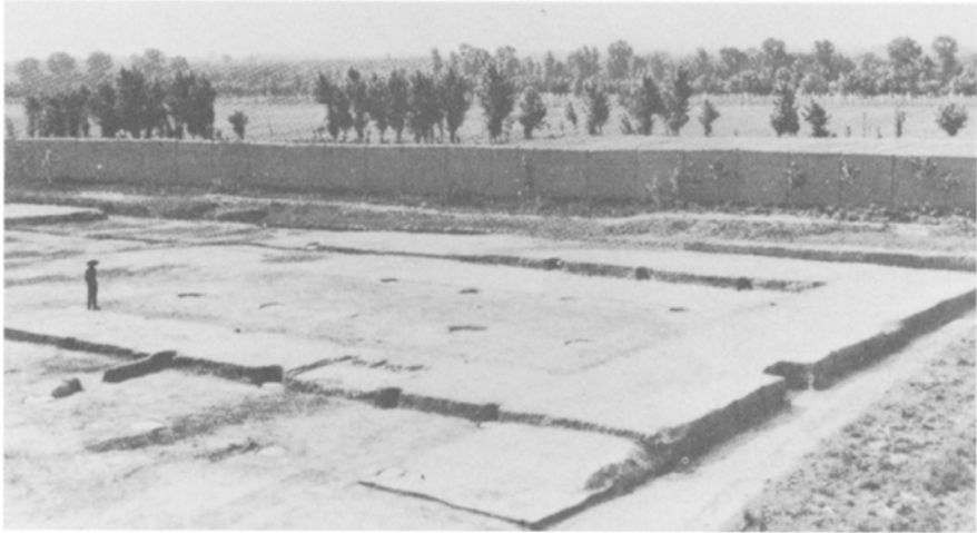
Fig. 6.2: View of footings from the southeast of the Wū Warehouse ( Wū kù 武庫), constructed in 198 BC in the Hàn dynasty capital of Cháng'ān 長安. Monochrome photograph taken by the excavation team in 1978. 725
